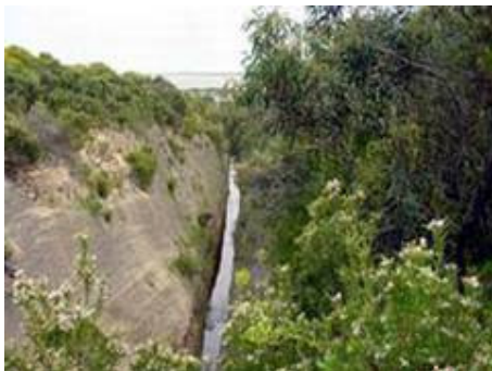
Woakwine Cutting, 1km long
